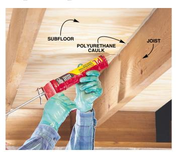
LOCATE the floor squeak and inject polyurethane caulk into gaps between the joists and plywood. Ventilate the area while using this caulk.
