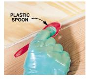
PUSH the bead of polyurethane caulk deeper into the flooring gap with a plastic spoon instead of your finger. This caulk is extremely sticky. Wear gloves when handling it and expect that any tools you use to work the caulk will have to be cleaned with paint thinner, or in the case of the spoon, just thrown away.
