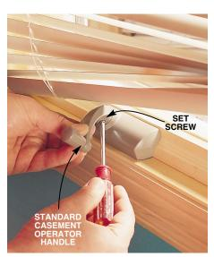
REMOVE existing standard casement window handles by loosening the set screw with a small straight-blade screwdriver. (This set screw also may be tightened to secure any loose window handle.)
