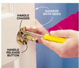
REMOVE the inside doorknob by locating the button (like our model), metal tab or wire clip on the side of the knob that acts as a release. Using an awl or small screwdriver, push the button in all the way—and at the same time—pull off the handle. Remove the door rose by inserting a small screwdriver into the small notch in the rose and twisting the tool to pop it off. Be careful so you don't chip any door paint.
